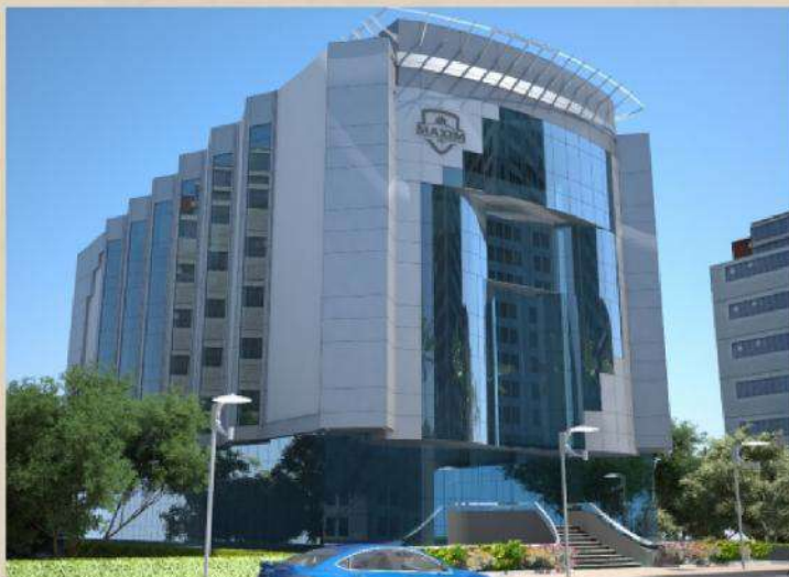
Maxim Building Admin Building
