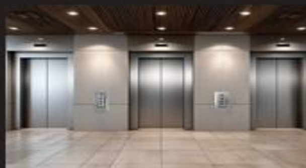
Multiple Elevators (passenger + service)
